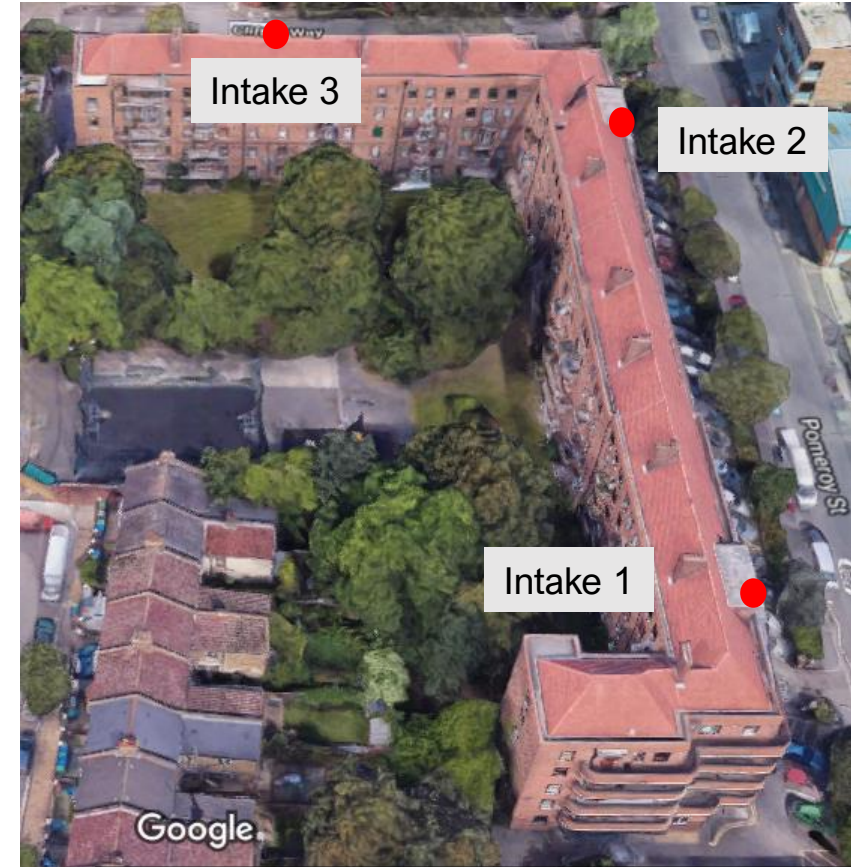
Fig 5. Location of electricity meters at Juniper House
