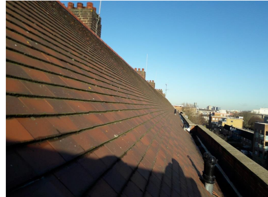
Fig 6. Terracotta roof tiles at Juniper House
